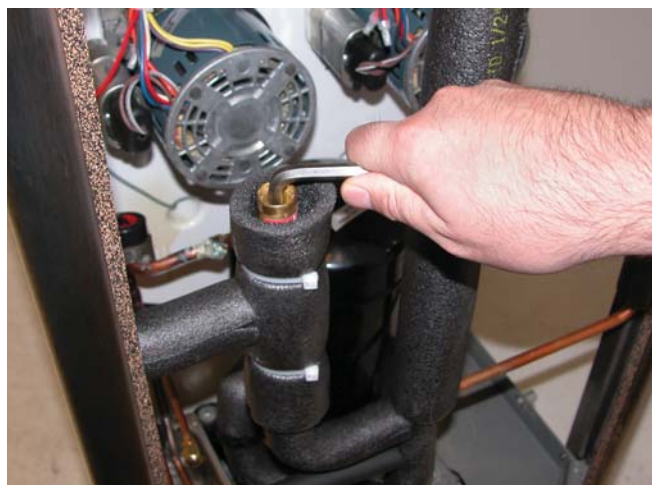
Figure 5-10 Hot Gas Bypass Adjustment
