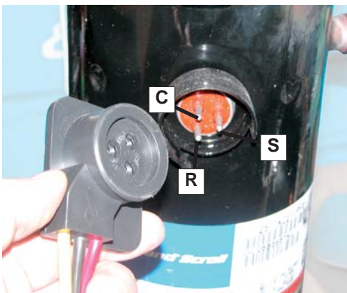
Figure 5-3 Compressor Connection
