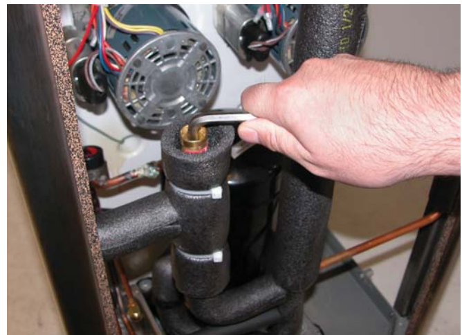
Figure 5-10 Hot Gas Bypass Adjustment
